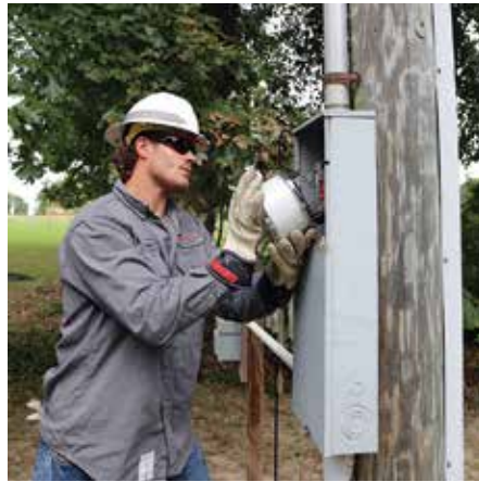
Southwestern Electric 3rd Step Apprentice Lineman Dawson Chesnut installs a new Advanced Metering Infrastructure (AMI) meter.
