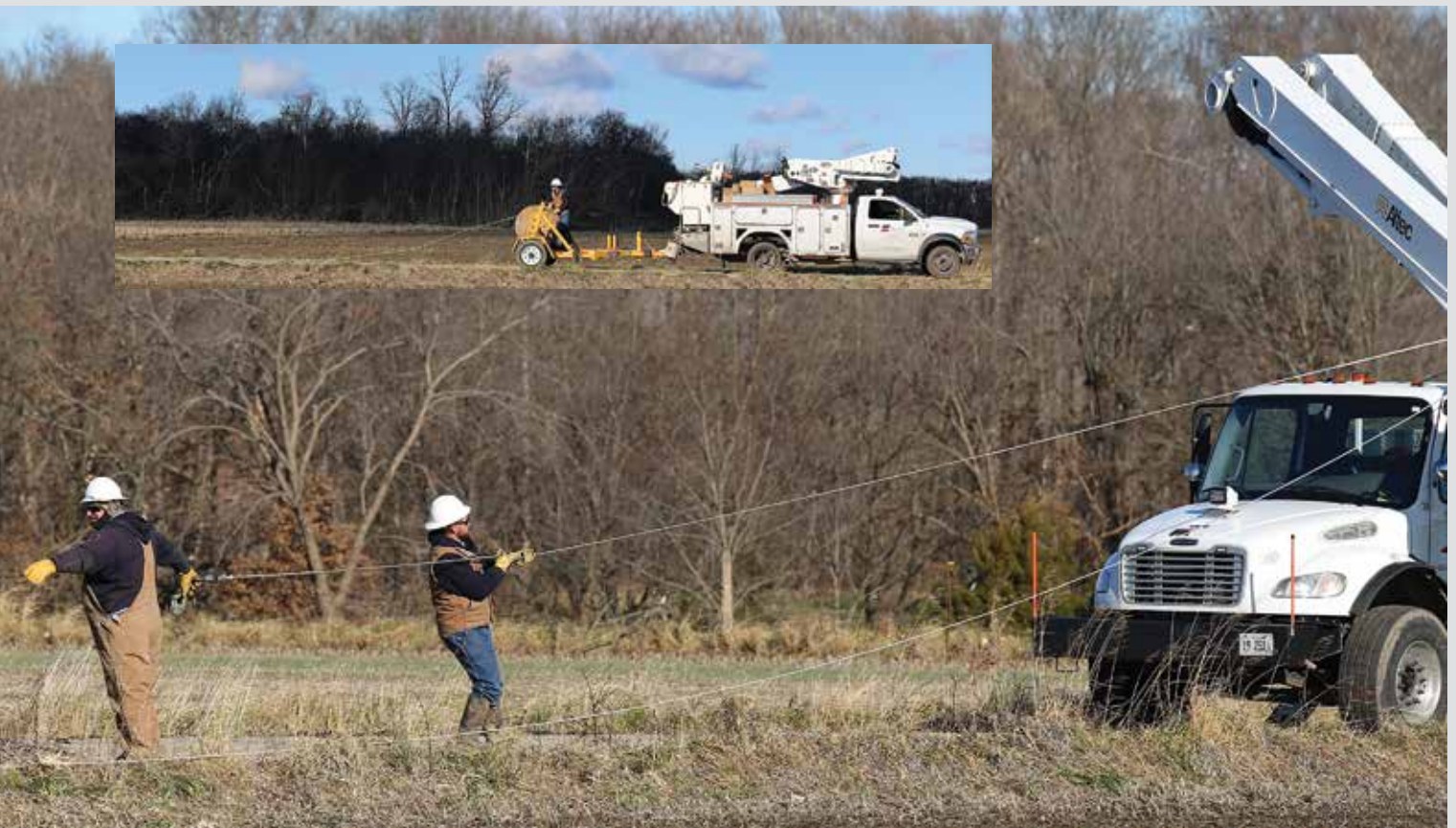
Rob Nesbit (left), maintenance foreman, prepares to attach new steel-reinforced aluminum conductor to a pole. Above: Storm debris lodges in a fallen tree. Below (l-r): Brian Bast, Rick Mersinger and Braden Clark (also in the inset) deploy new conductor east of Highway 51. Bast and Clark are journeymen linemen and Mersinger is a Southwestern Electric maintenance foreman.
