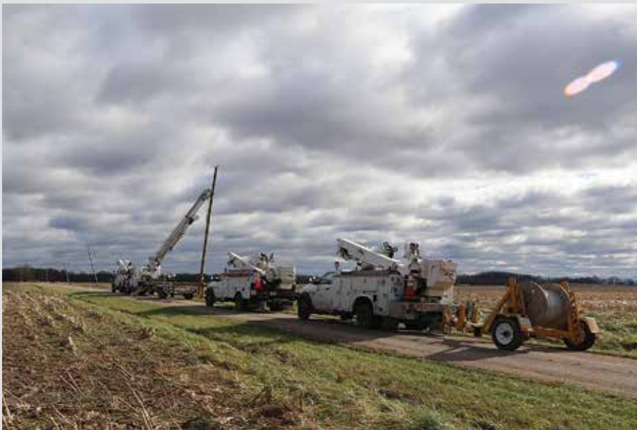
Crews work in frigid winds to repair tornado-damaged lines along a Fayette County road (above) and Highway 51 (below). Rick Mersinger (upper right), maintenance foreman, guides a new pole into position using a remote.
