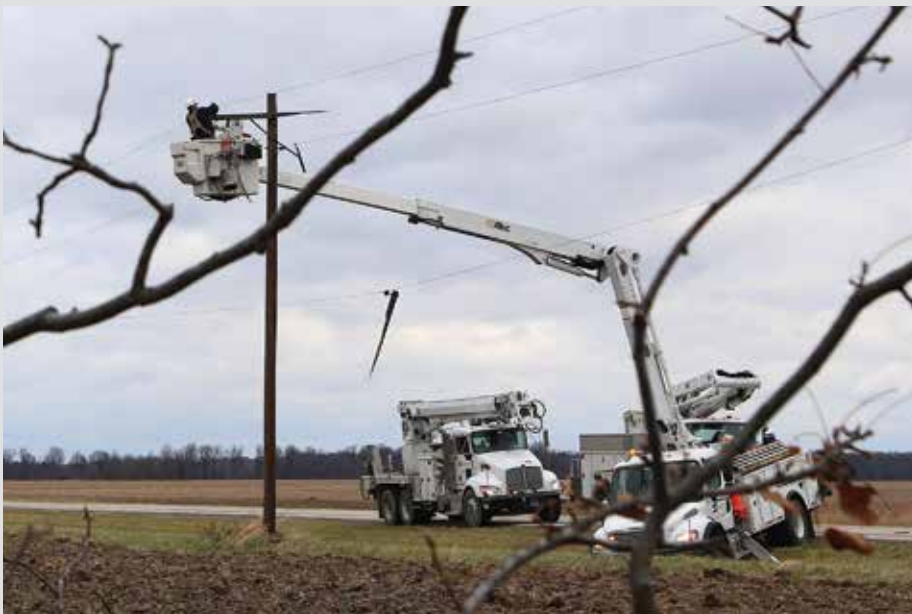
Crews work in frigid winds to repair tornado-damaged lines along a Fayette County road (above) and Highway 51 (below). Rick Mersinger (upper right), maintenance foreman, guides a new pole into position using a remote.
