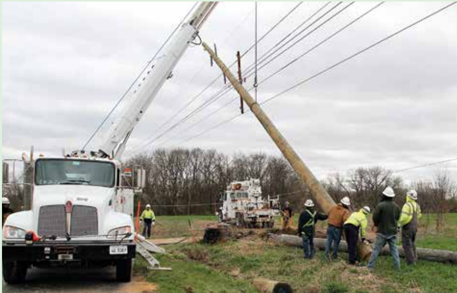
Crews place a new transmission pole. Pictured at right are (l-r) Southwestern Electric's Tyler Meseke, journeyman lineman; Kyle Hails, maintenance foreman; Ethan Fulk, journeyman lineman; and DJ Haarmann, construction foreman.
